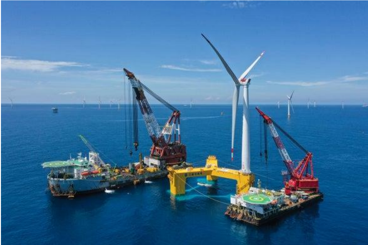
Offshore support vessels constructing an offshore wind farm in Yangjiang, Guangdong Province, China. Credit Liang Wendong, Getty Images
